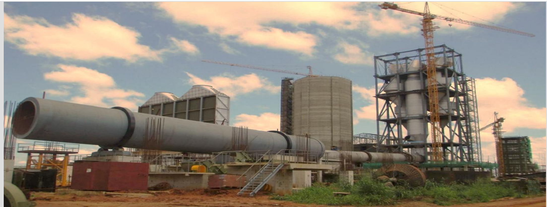
Scantogo clinker plant construction (Togo)
